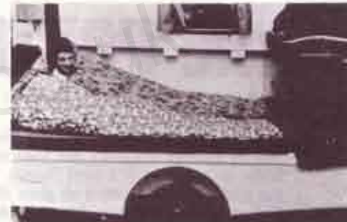
6. This mock-up shows sleeping arrangements for four people. Normally, the two transverse bunks are supported by the walls of the van.
